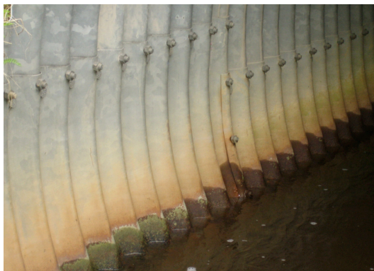
Figure 2. Typical rust in water line after 30 years
