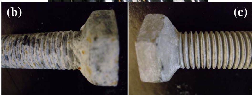
FIGURE 4 (a) Example of staining in the obvert of a structure coated with the thermoplastic polymer system. (b) Galvanized bolt following removal from test chamber compared to (c) duplex coated bolt at three times the exposure time.
