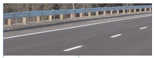
Guiderail is manufactured to the highest specifications (AASHTO M180-78) from 2.5 mm steel. All componenets, including nuts and bolts, are hot dip galvanized in a process (CSA G-164M) that provides double the zinc protection of pregalvanized steel. This ensures long service life for all applications.
