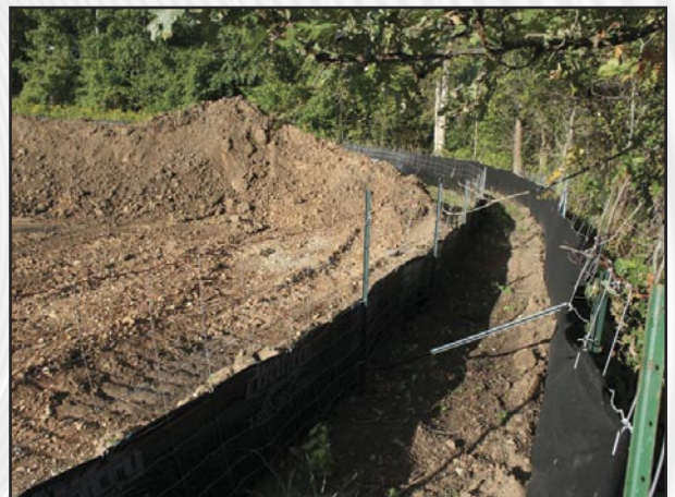
SEDIMENT AND EROSION CONTROL FENCE PROTECTING WETLANDS AT HCBP DURING CONSTRUCTION
