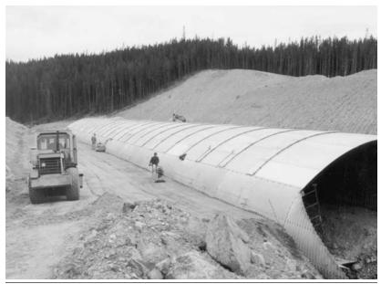
Backfill proceeds parallel to structure.
