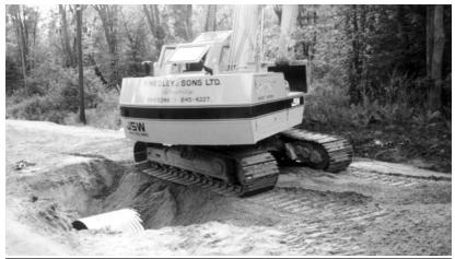
Construction load on pipe.
