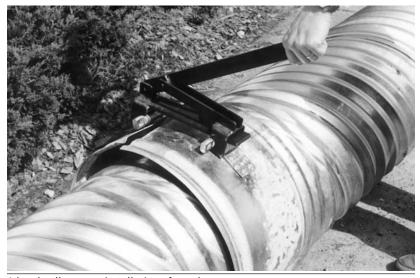
A band puller eases installation of coupler.
