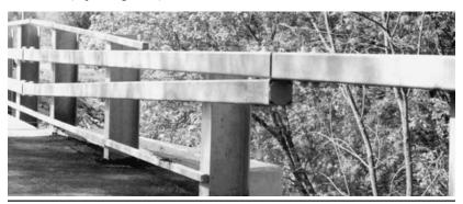
Transition from bridge rail to box-beam guiderail.
