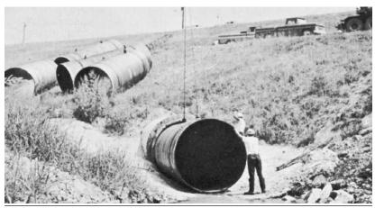
Sliplining a concrete culvert with steel pipe.
