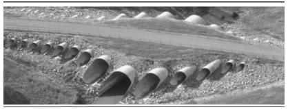
Combination stream crossing and voids to reduce dead load on foundation soils. (Ontario Ministry of Transportation project.)
