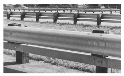
Offset mounting of W-beam on wood post.
