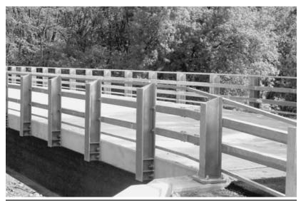
Typical bridge tubular steel railing.
