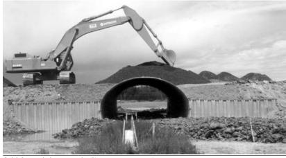
Cold-formed sheet steel piling prevents erosion.
