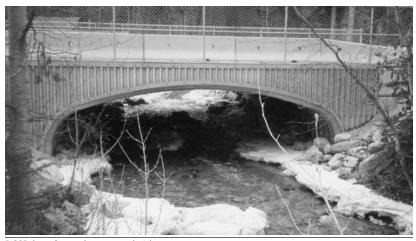
DCSP box for a short span bridge.
