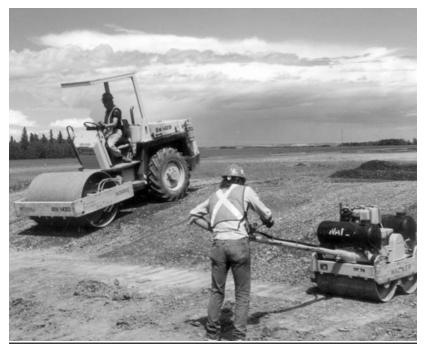
Backfill compaction over long span proceeds in a direction perpendicular to the length of the structure.
