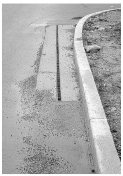
CSP slotted drain inlet.
