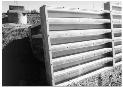
Face of bin type retaining wall.
