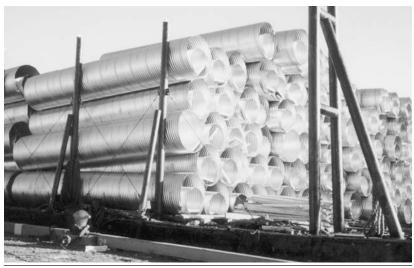
CSP for storm drainage project.
