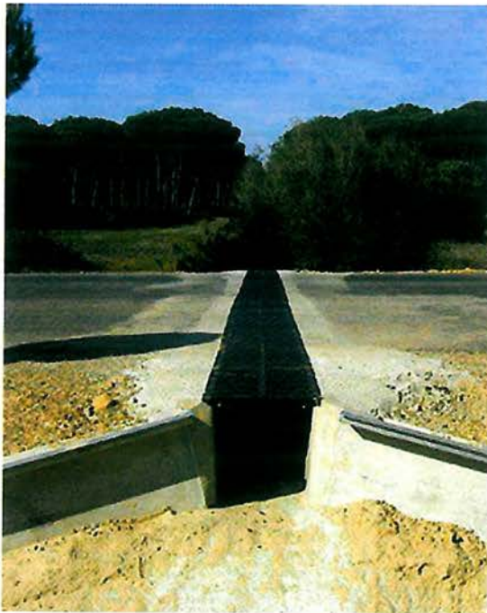
Figure 7.74 - Amphibian tunnel with open grid in Spain. (Photo by Giasa, Spain)
