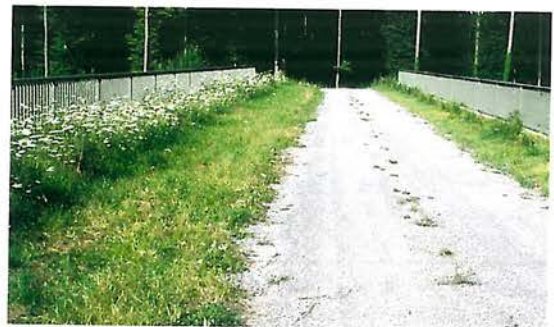
Figure 7.32 - A vegetated strip alongside a forestry track can enhance the permeability of infrastructure for small animals. A bridge across the high-speed railway line near Oberderdingen in Germany. (Photo by B. Georgii)
