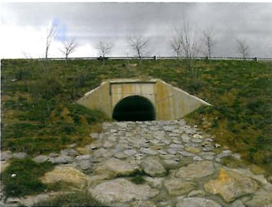
Figure 7.64 - Stepped exits of drains are traps for small animals (top). The two exits in Spain (centre, bottom) have been adapted so that animals passing through the drainage culverts do not get trapped. (Photos by C. Rosell)
