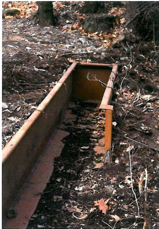
Figure 7.71 - A U-shaped end of the fence forces amphibians to turn back and reduces the number of animals continuing onto the road at the end of the fence. (Photo by S. Zumbach)
