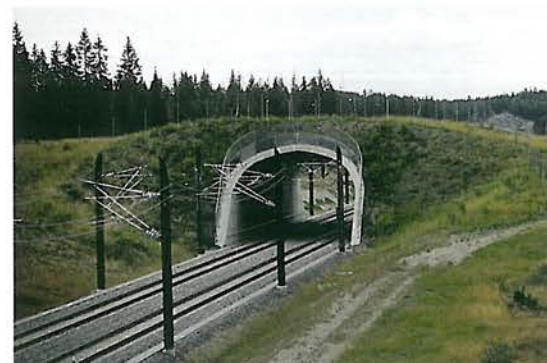
Figure 7.25 - A wildlife overpass across a high-speed railway line in Norway (44 m wide) preserving an important migration route of moose. (Photo by L. Kastdalen)
