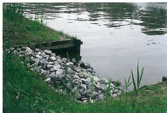
Figure 7.96 - Different possibilities for fauna exits on waterways in the Netherlands. Exits at the water side of the sheet piling is only possible when there is no danger for ships. In use by badgers, roe deer, young ducks and hedgehogs. (Photos by H. Bekker)
