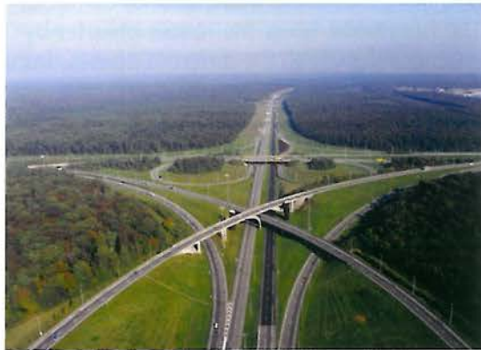
Figure 1.1 - Transport infrastructure can fragment habitats, as with this example at the A36 interchange, Alsace, Forest of Hardt (Haut-Rhin), France. (Photo by J. Carsignol)
