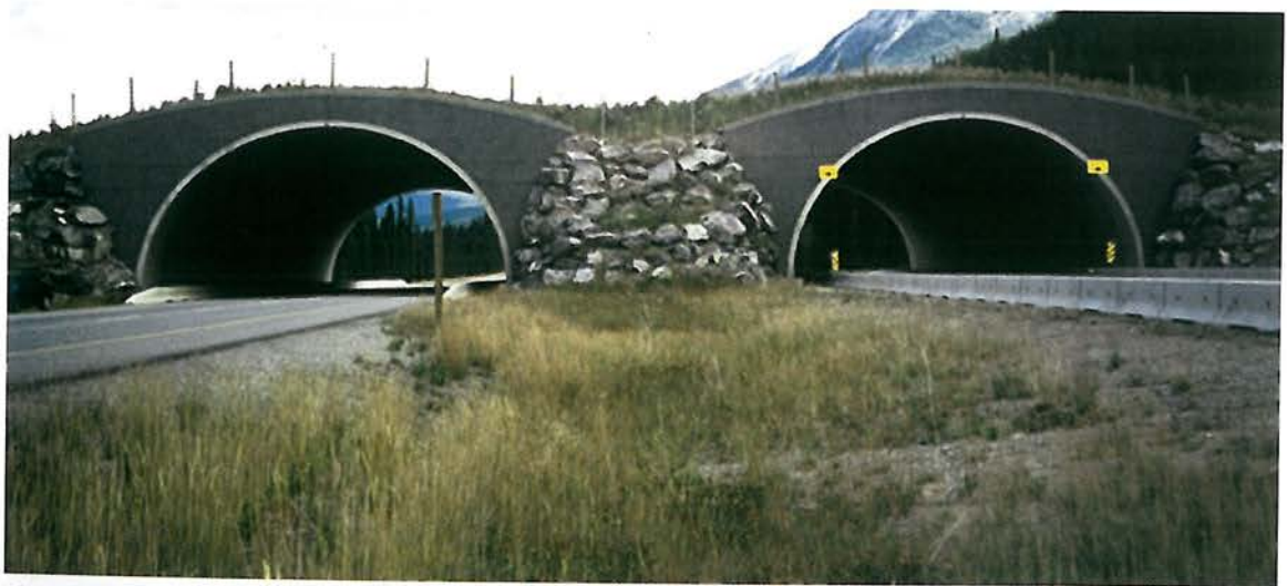
Figure 7.19 - This wildlife overpass in Banff national park on the Trans Canada Highway was built with prefabricated elements across an existing road. (Photo by H. Bekker)
