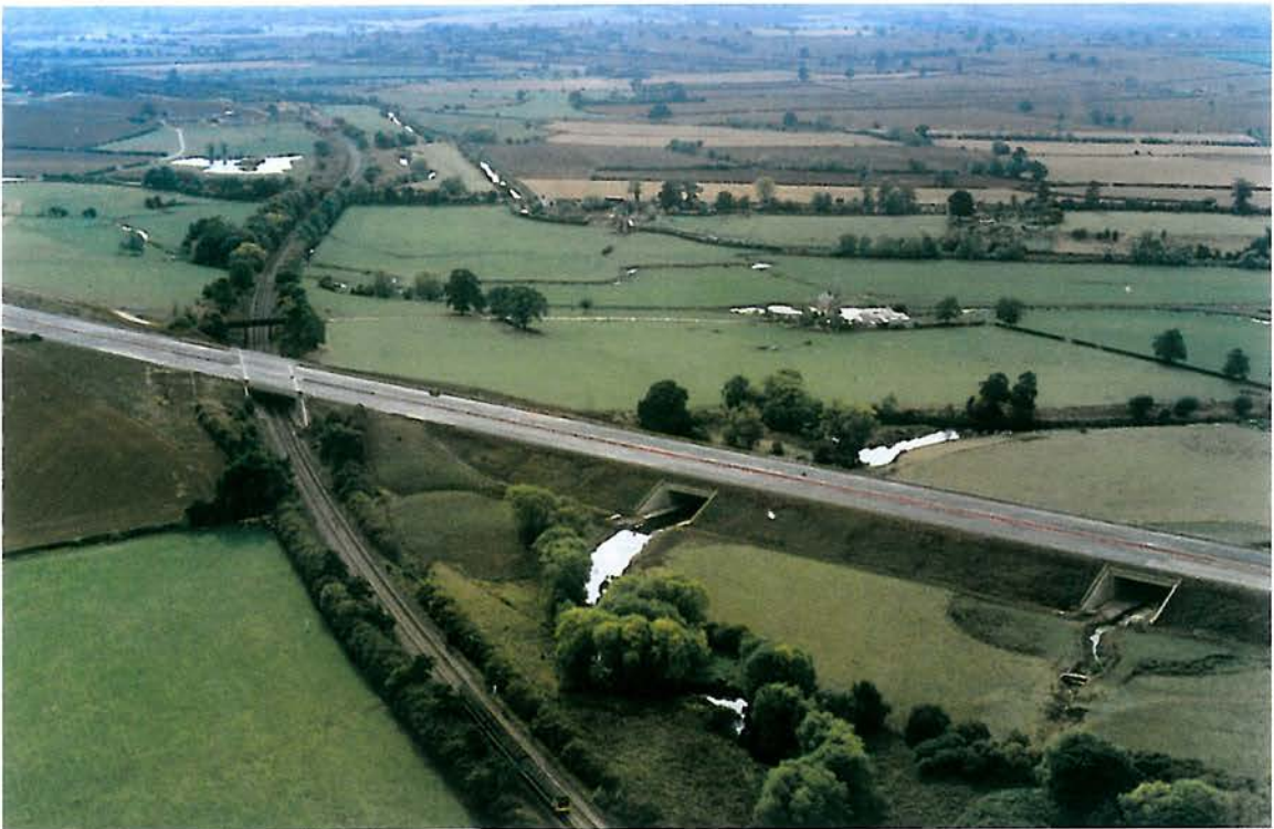
Figure 6.5 - M40, Cherwell Valley, Oxfordshire. The embankment is a dominant feature but care has been taken to retain the character and form of the river on both sides of the road. (Photo by Highways Agency, UK)
