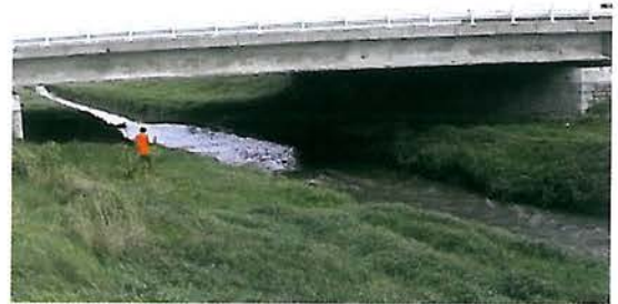
Figure 7.48 - If bridges over streams are built wide enough to preserve the natural banks of the river, they can be used as underpasses by animals, like in this example from the Czech Republic. (Photo by J. Dufek)
