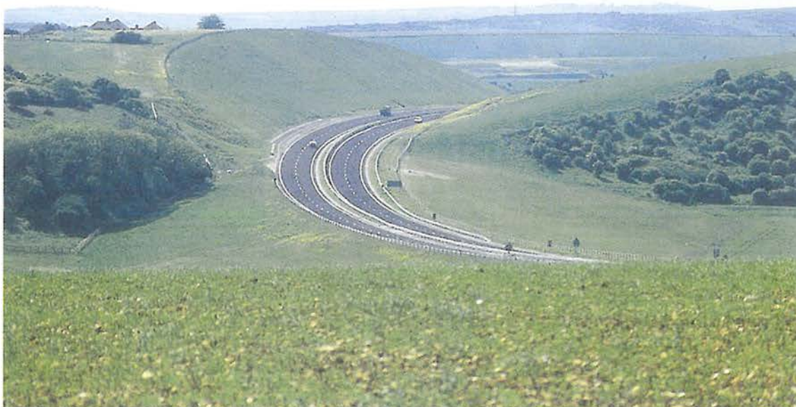
Figure 6.2 - The A27 Brighton bypass runs through the edge of the South Downs AONB in Southern England. Grading the cuttings and embankments to 1:6 fits the road into the downland character. (Photo by Highways Agency, UK)
