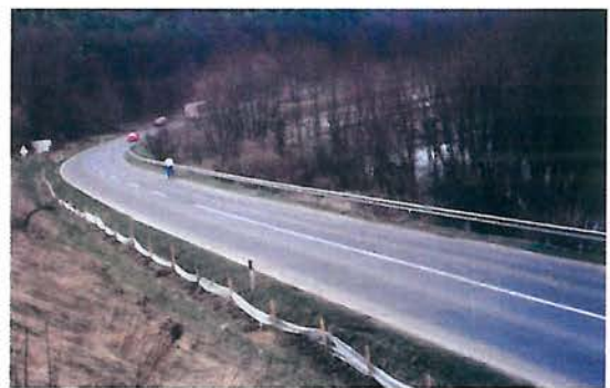
Figure 7.70 - A strong opaque plastic foil can be put up without stabilising wire mesh, as in this example from Hungary. However, the posts should not be placed on the side the amphibians approach from to improve the guiding function of the fence. (Photo by M. Puky)
