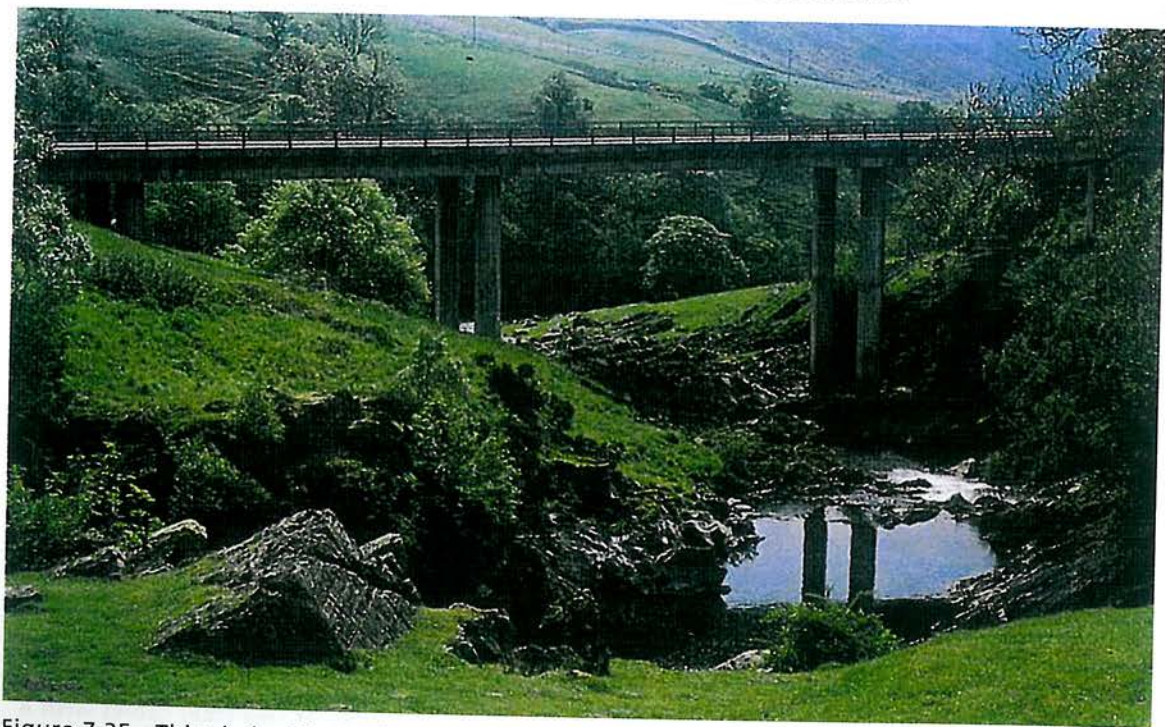
Figure 7.35 - This viaduct in northern England leaves the river valley intact. (Photo by Highways Agency, UK)
