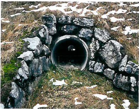
Figure 7.54 - Entrance to an underpass for small animals at the A8 in Switzerland (diameter 1 m). Stone walls, which in this mountain region are a common feature, guide animals to the passage. (Photo by A. Righetti)
