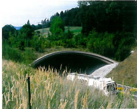
Figure 7.11 - The overpass Schwarzgraben in southern Germany (B31neu, 50 m wide, combined with local road) is densely covered with bushes and small trees since it aims at connecting the adjacent forests. (Photo by V. Keller)
