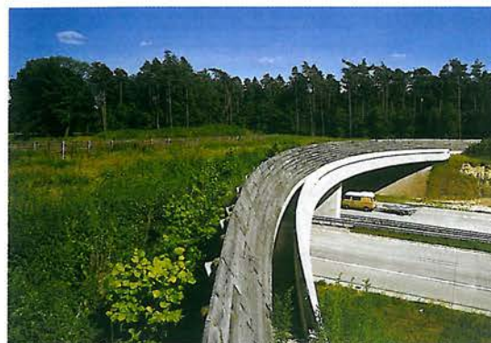
Figure 7.14 - The example of the Boerskotten wildlife overpass (the Netherlands) shows a screen made of wood. The screens have to be as close to the outer edge as possible to ensure a maximum width for wildlife. The ledge on the outside is designed to allow safe access for maintenance. (Photo by H. Cormont)
