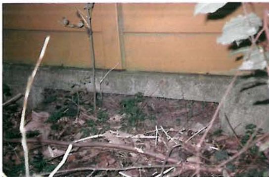
Figure 7.90 - This noise barrier has openings at the bottom to reduce the barrier effect for small animals. (Photo by H. Bekker)
