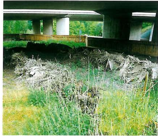
Figure 7.42 - Tree stumps were used as shelter for animals under the Zandheugel viaduct on the A27 in the Netherlands. The screen which separates the road from the stump walls can be seen in the background. (Photo by H. Bekker)
