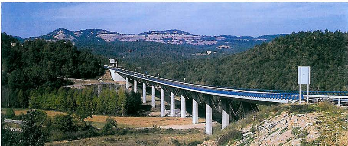
Figure 7.38 - This large viaduct in Spain (road C25 near the Natural Park of Montseny) shows different zones under the viaduct: roads, natural vegetation, etc. Spatial planning has to ensure that the parts suitable for the passage of animals remain so in the long term. (Photo by C. Rosell)
