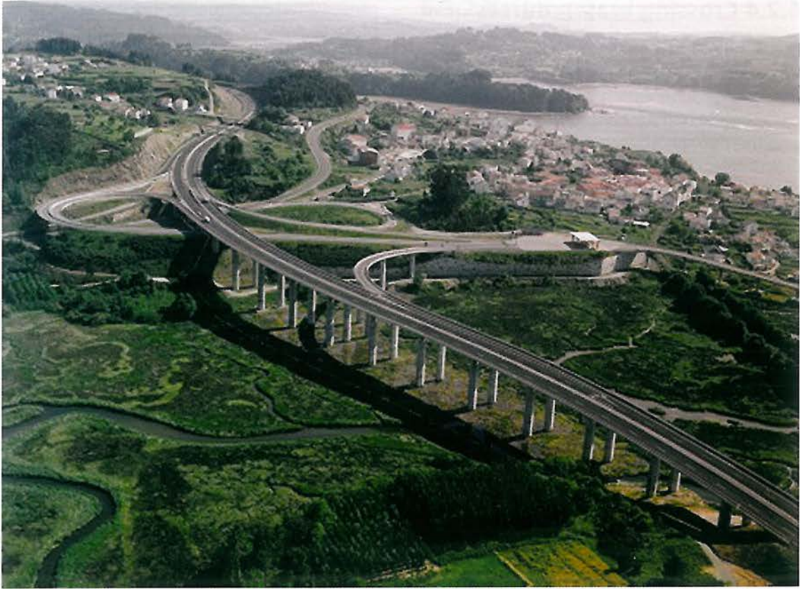
Figure 6.4 - Viaducts minimise landtake and fragmentation within a valley by allowing watercourses and any existing nature conservation interests to continue under the structure. This viaduct carries the A9 highway over an important wetland surrounding the River Mino (Galicia, Northwest Spain). (Photo by AUDASA, Spain)
