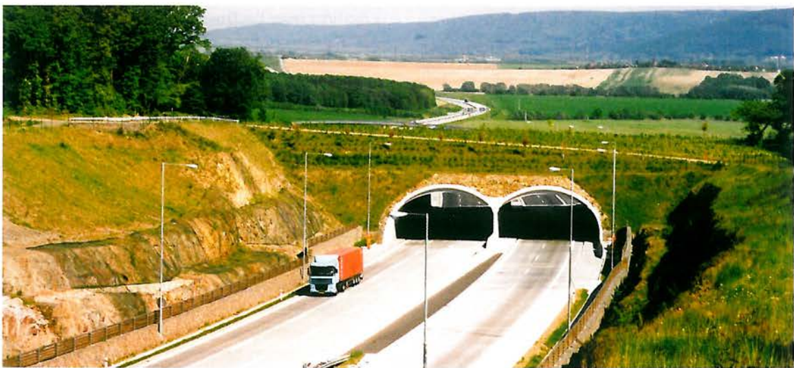
Figure 4.4 - Mitigation measures can be used to reduce the barrier effects of infrastructure. This is an overpass near Lipnik nad Bécvou, Czech Republic, frequently used by a range of species including roe deer and wild boar. (Photo by V. Hlaváč)
