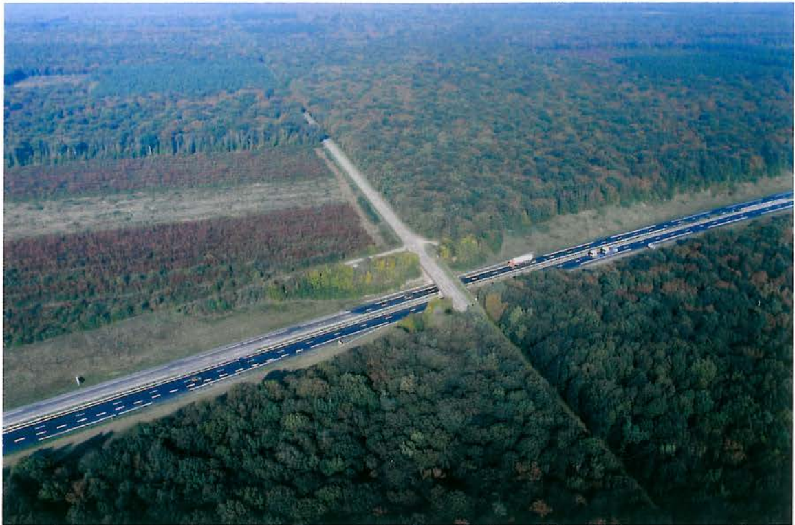
Figure 4.2 - Transport infrastructure can fragment habitats, like here at the A36 motorway, Alsace, France. This is an intersection with a minor road leading to fragmentation of the forest environment (Forest of La Hardt). (Photo by J. Carsignol)
