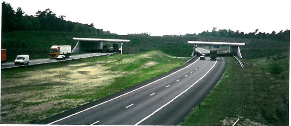
Figure 7.18 - The wildlife overpass Harm van der Veen (Kootwijk, the Netherlands) was built in 1998 over two separate parts of the motorway A1. This was a significant milestone, because it was the first overpass in the Netherlands to be built across an existing motorway. (Photo by H. Bekker)
