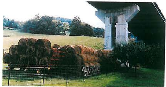
Figure 7.40 - In this example of the RN59 in France, the function of a viaduct to preserve movement of animals is lost, since access is blocked both by a fence and by stored material. (Photo by J. Carsignol)
