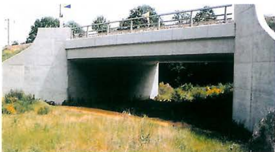
Figure 7.45 - This underpass is below a high-speed railway line in France and has a good openness index, suitable for large mammals. (Photo by SETRA)
