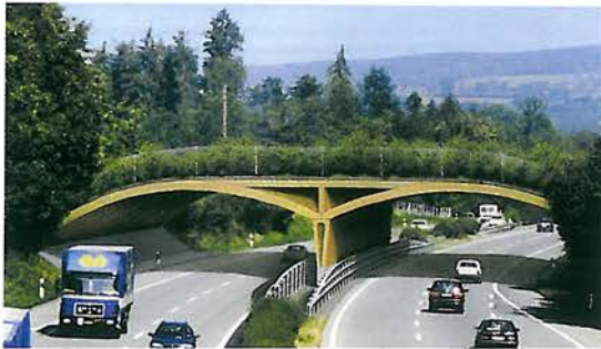
Figure 7.26 - Until now, overpasses constructed with wood have rarely been built. At one overpass in France problems arose due to high maintenance costs. This photomontage from Switzerland shows what a modern construction of a wooden overpass could look like. (Illustration by Marbach & Marbach, Eich, Copyright Swiss Ornithological Institute)
