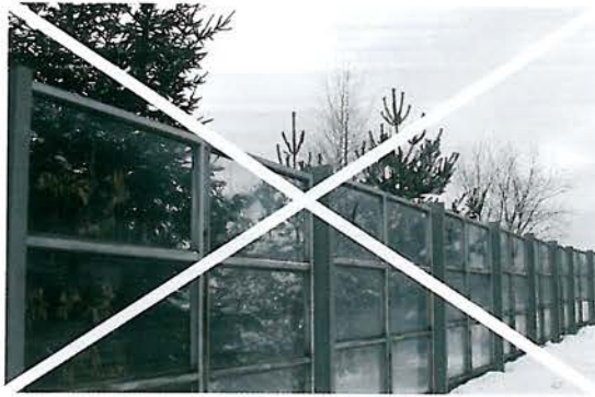
Figure 7.93 - The planting of bushes close to transparent screens should be avoided. (Photo by V. Hlaváč)
