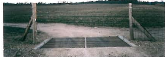
Figure 7.84 - Cattle grids are usually used on agricultural tracks as in this example from Denmark. However, they can also be used where a side road enters a main road. (Photo by B. Wandall)
