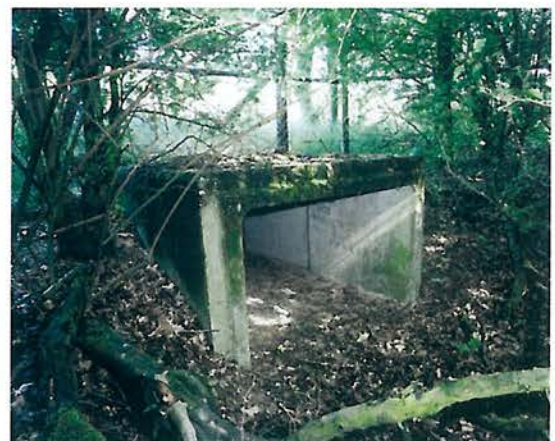
Figure 7.53 - A rectangular underpass for small animals, (1.2 m wide, 0.8 m high and 40 m long; A50 near Hernen, the Netherlands). This underpass is often used by badgers. (Photo by H. Cormont)
