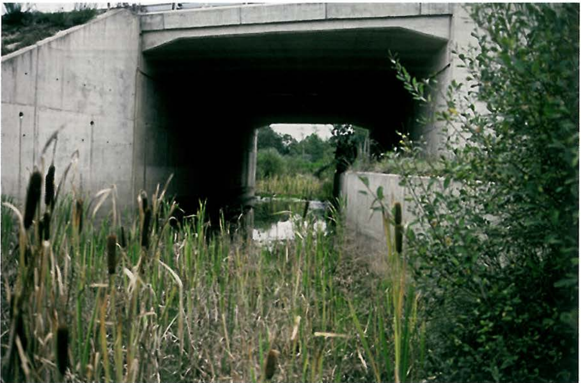
Figure 7.51 - The main purpose of this underpass at the A10 in France is water management in a wetland. The dimensions and the integrated ledge allow movement of small and medium-sized mammals. (Photo by H. Bekker)
