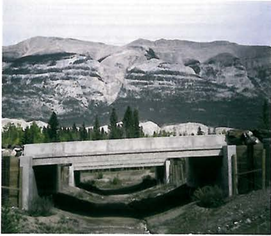
Figure 7.41 - In Banff National Park (Canada) two parallel structures were constructed to minimise the length of the underpass and to provide increased light below. (Photo by H. Bekker)
