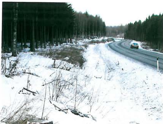
Figure 7.89 - Cutting high vegetation alongside the roads makes large mammals, e.g. moose like in this example from the E18, Akershus in Norway more visible to drivers, and removal of vegetation which is an attractive food-source will reduce the risk of having animals foraging along the road. (Photo by B. Iuell)
