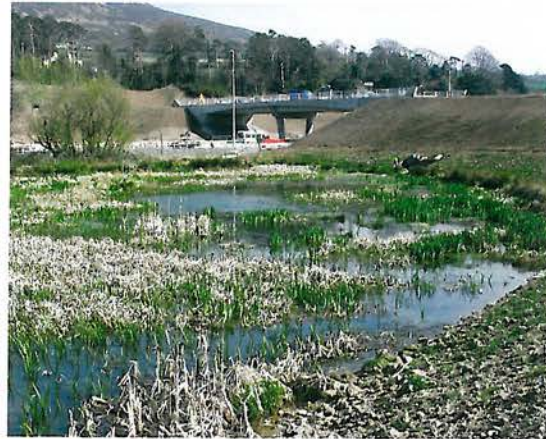
Figure 8.3 – Example of wetland construction in the Glen of the Downs, Ireland. Above: during construction, below: on completion. (Photo by R. Nairn)
