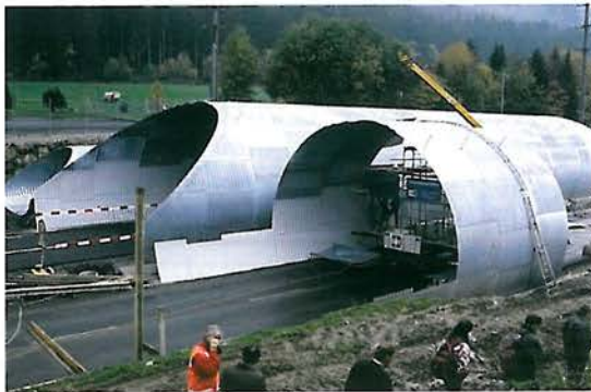
Figure 7.22 - Corrugated steel elements were used for the overpass Schindellegi in Switzerland (40 m wide), which was constructed across an existing road which was widened. This allowed traffic flow along one lane during the whole of the construction phase. (Photo by O. Holzgang)
