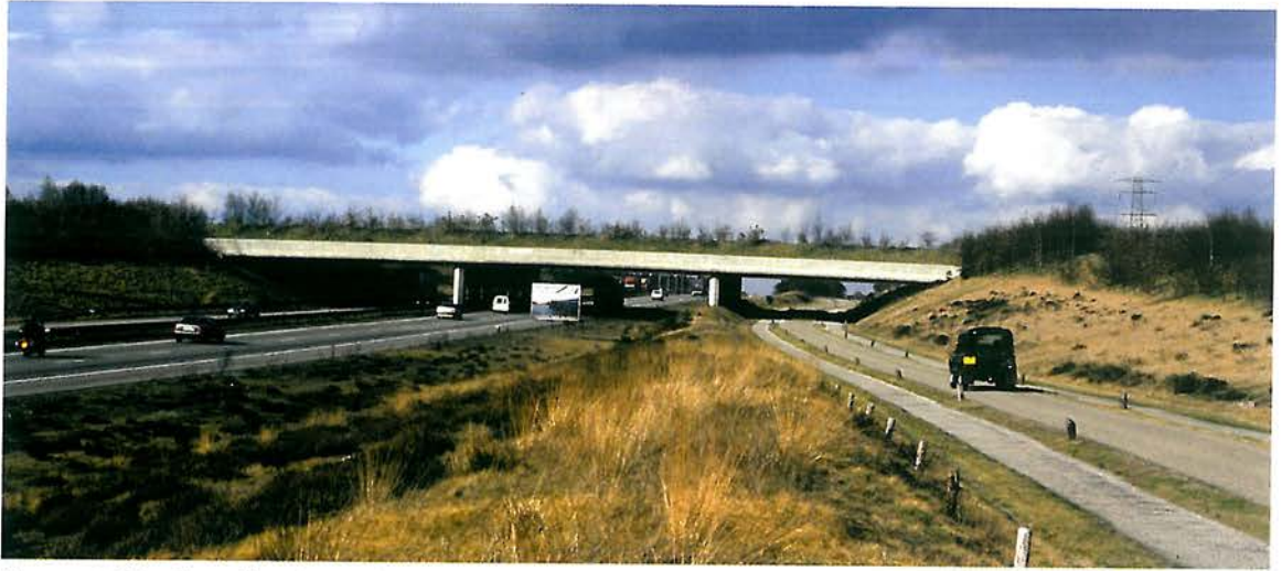
Figure 7.17 - The side view of Terlet north of Arnhem (the Netherlands) shows a straight concrete construction on pillars. The road level has been lowered to allow the overpass to cross at the level of the adjacent land. (Photo by V. Keller)
