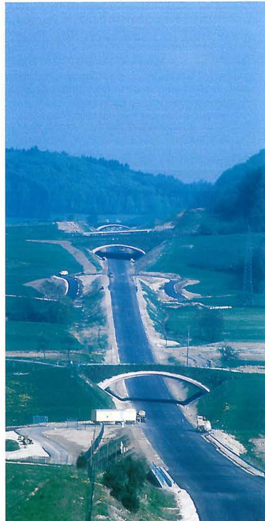
Figure 7.7 - The three-lane highway B31n in Southern Germany cuts off an area along Lake Constance. A high density of passages prevents the habitats from becoming isolated. Passages include wide wildlife overpasses as well as narrower ones combined with agricultural and forestry tracks. (Photo by V. Keller)
