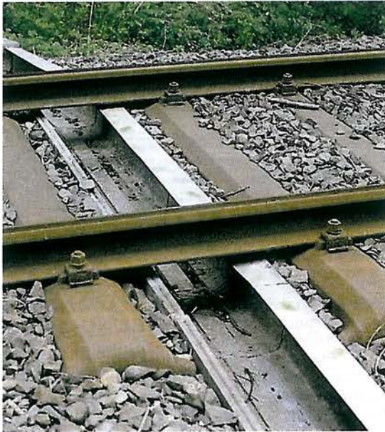
Figure 7.76 - For amphibians and other small animals, half-pipes can be used as passages under the rails where larger tunnels are not possible. (Photo by U. Bolz)
