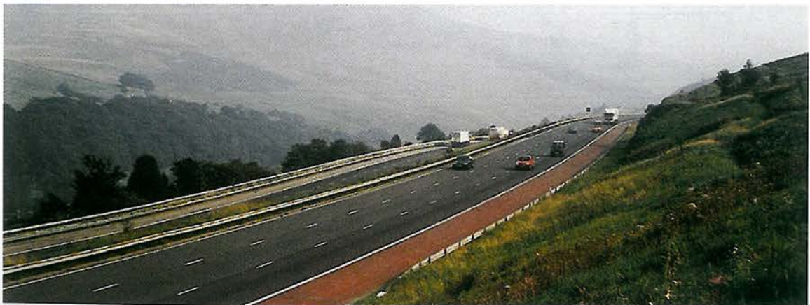
Figure 6.3 - M6, Cumbria in Northern England. The road follows a major ridge and avoids the river valley. Verges are restored to the classic upland vegetation types. (Photo by Highways Agency, UK)
