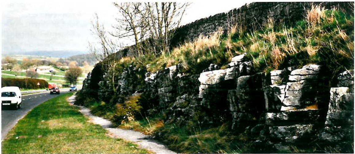
Figure 6.7 - A6, Derbyshire. This rock outcrop, where naturally regenerated vegetation has become established and the characteristic form of the limestone is exposed, gives a very distinctive character to the road. The dry stone wall emphasises the outcrop. (Photo by Highways Agency, UK)
