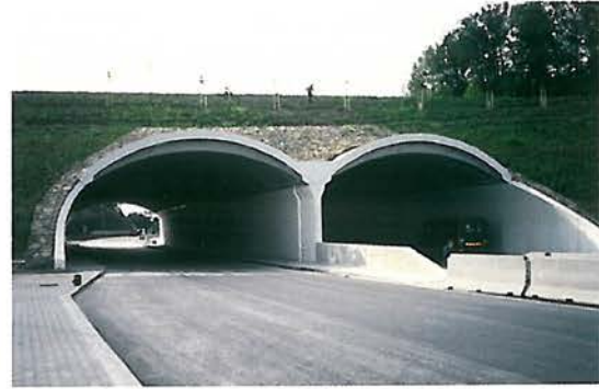
Figure 7.21 - Wildlife overpass in the Czech Republic with two prefabricated arches made of concrete. (Photo by H. Bekker)
