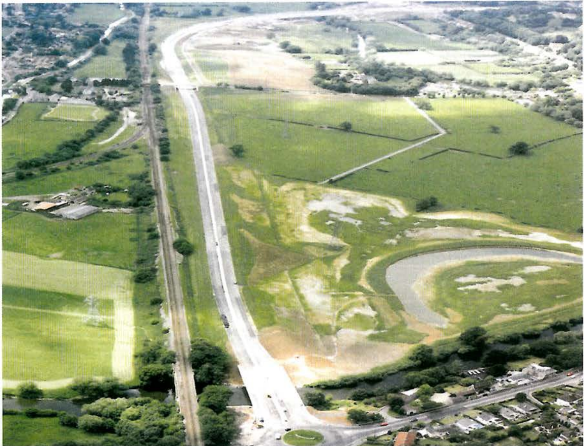
Figure 6.1 - A4/A46 Batheaston/Swainswick bypass - within the Cotswolds Area of Outstanding Natural Beauty (AONB) and adjacent to the World Heritage City of Bath, UK. Landscaping was developed with highway design to ensure the best possible fit with the landform. There was extensive use of false cuttings and shallow embankments to screen traffic and blend the engineering slopes gently into the landform. (Photo by Highways Agency, UK)
