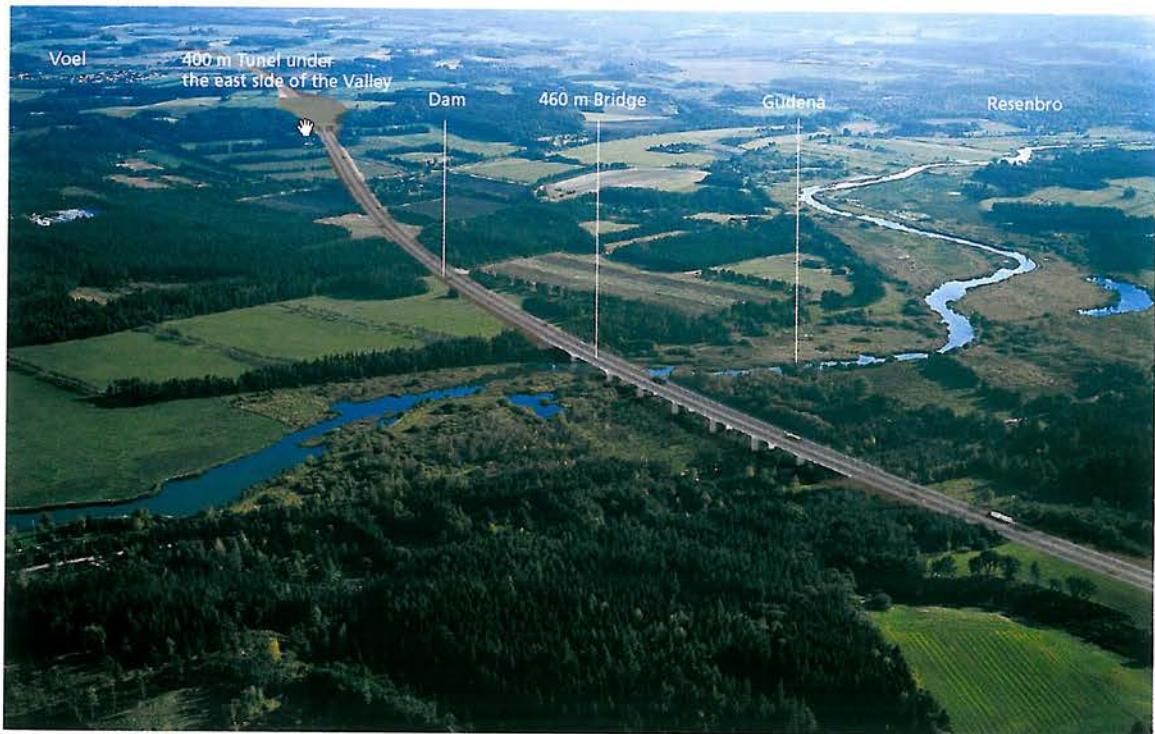
Figure 5.6 and 5.7 - Computer visualisations showing alternative options for a viaduct crossing the Gudena river valley, Denmark. (Danish Road Directorate: VVM Motorvejen Herning-Århus ved Silkeborg)
