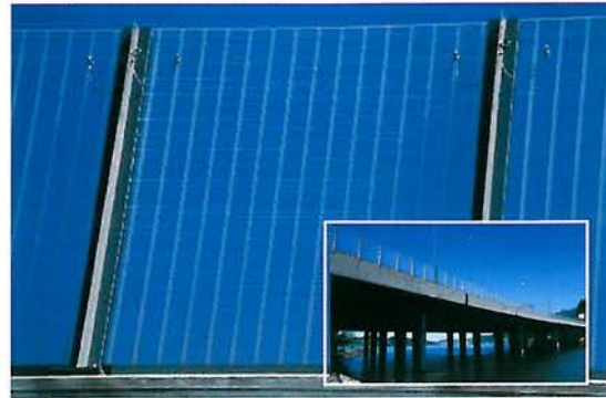
Figure 7.91 - Transparent noise barrier along a motorway in Switzerland with vertical markings. (Photo by H. Schmid)
