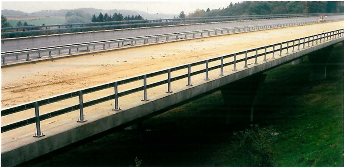
Figure 7.37 - A long viaduct on a slope as opposed to an embankment preserves the habitat and allows animals to move freely, as with this example of a Swiss motorway. (Photo by H. Bekker)
