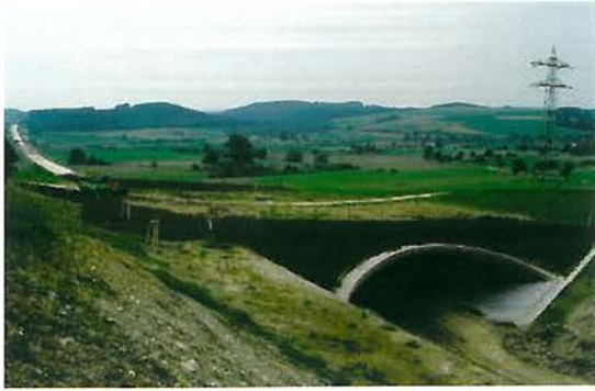
Figure 7.20 - The shape of the 80 m wide landscape bridge Hirschweg (B31neu, southern Germany) takes up the slope of the hill and leads animals across the road, which has been placed in a cutting. The picture was taken before the bushes planted as screens had grown. Nevertheless the overpass was intensively used by mammals as soon as it was covered with earth. (Photo by V. Keller)
