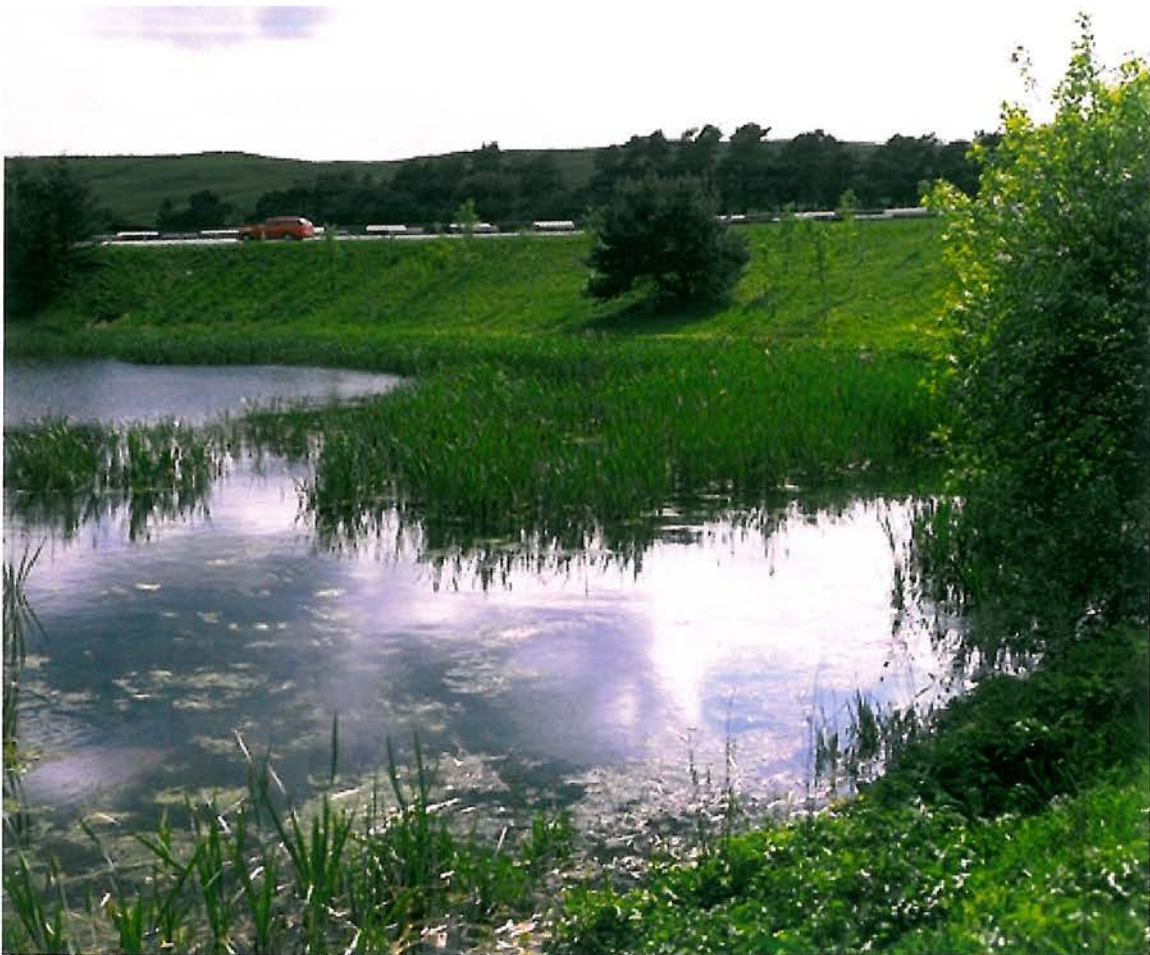
Figure 6.11 - Balancing ponds provide an opportunity to create features of landscape and wildlife interest. (Photo by Highways Agency, UK)
