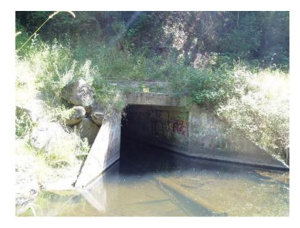
FIGURE 7- This concrete box culvert at Deadman Creek on US 2 was considered a barrier due to excessive water
