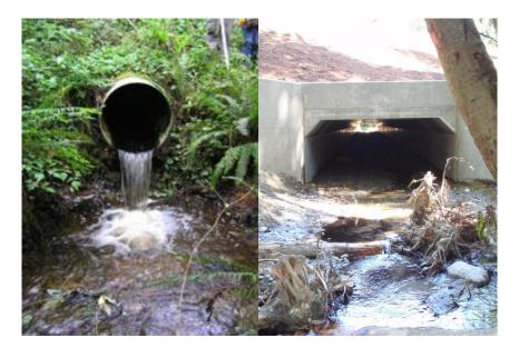
FIGURE 3- A 0.7 m (2.2 ft) round culvert was replaced with stream simulation designed 3.6 m (11.8 ft)
