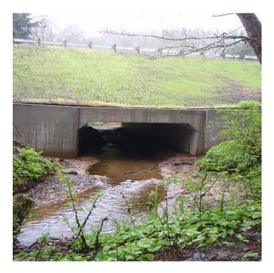
FIGURE 4- A round culvert was replaced with stream simulation designed 4.9 m (16 ft) span x 2.9 m (9.5 ft) rise
