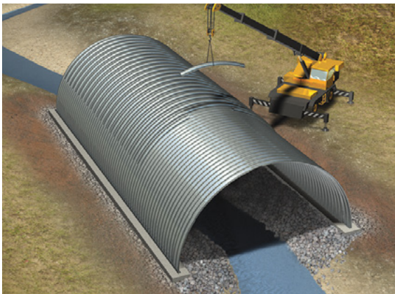
If specified, reinforcement ribs are then added.
