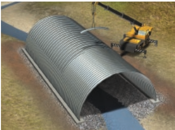
If specified, reinforcement ribs are then added.
