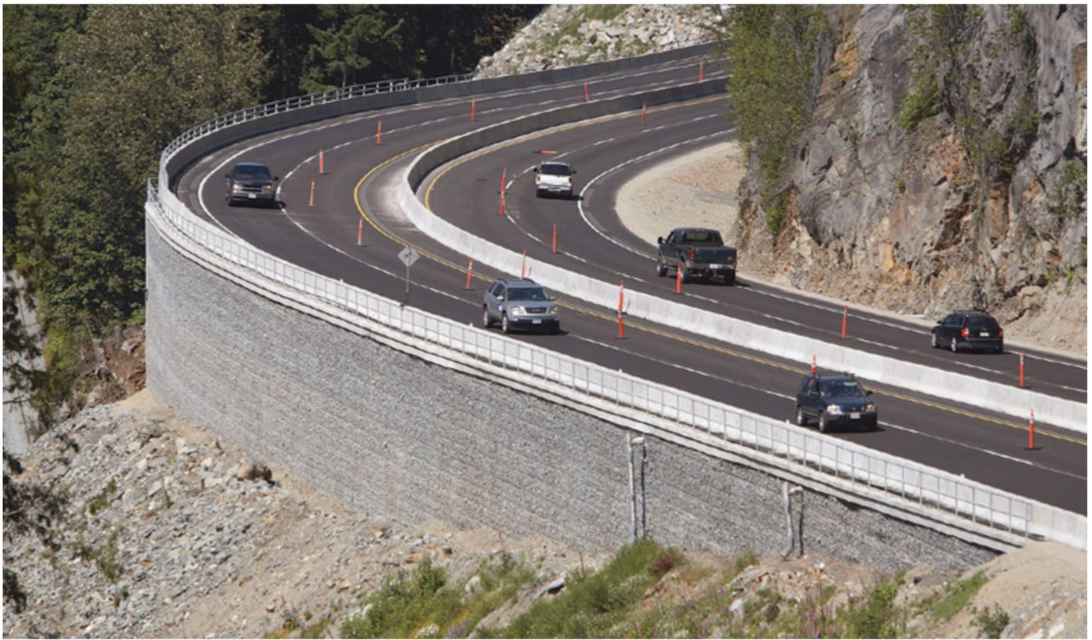
Wire Walls use cost-saving wire components and native backfill materials wherever possible.
