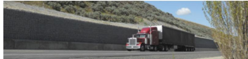
They easily accommodate curves, angles, or steps and the facing and soil reinforcing systems allow for the installation of culverts, bridge piles, or other site requirements.
