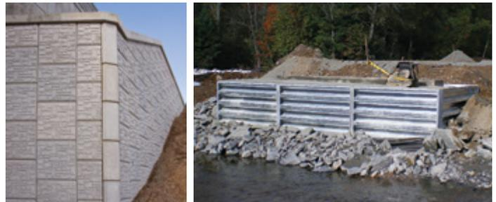
AIL offers various types of economical and easy-to-install abutment systems, including MSE structural walls (precast concrete panel or wire at the face) and Bolt-A-Bin® cellular bin style retaining walls. **See pages 28-33 and 36**
