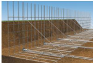
Backfill added over first course of reinforcement.
