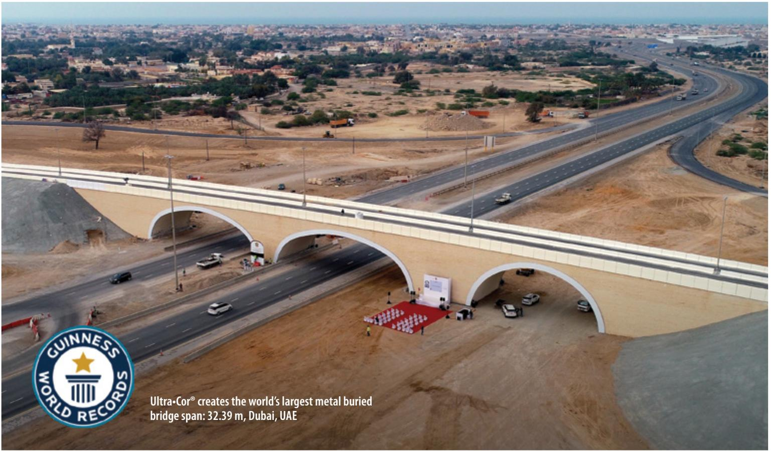
Ultra-Cor® creates the world's largest metal buried bridge span: 32.39 m, Dubai, UAE
