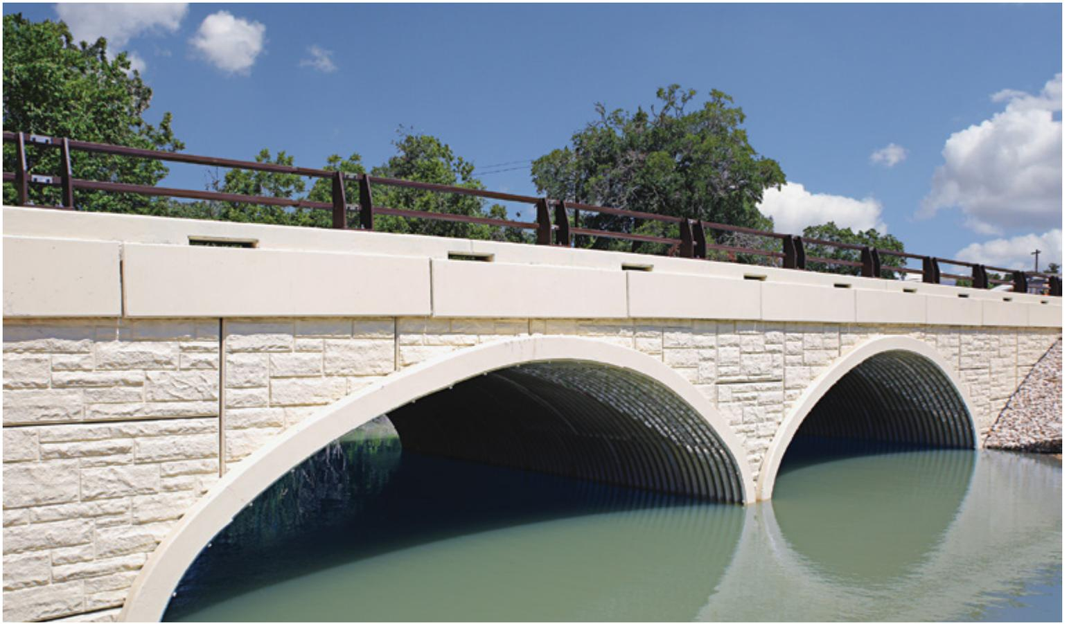
Corrugated metal structures ship and assemble easily in all seasons and in remote locations, often without the need for concrete.
