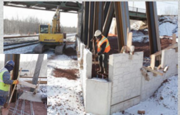
Leveling pad is installed on a compacted base.
