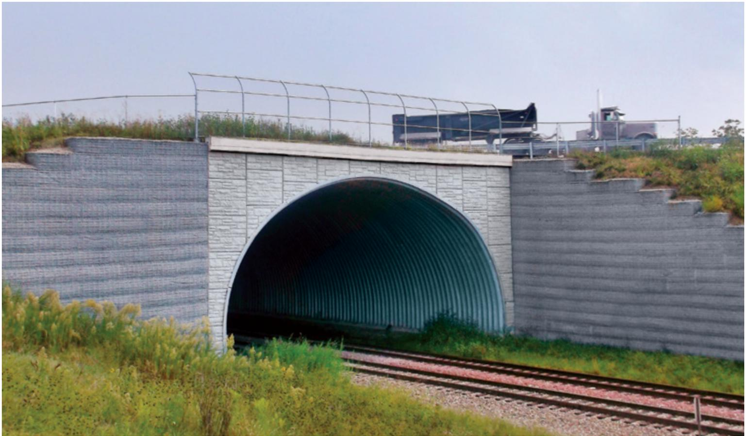
Lightweight and super strong, Super-Cor® is the most internationally-accepted and widely-used deep corrugation profile.
