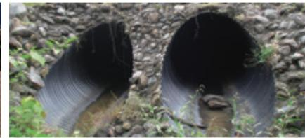
It will not crack under impact loads or vibrations due to the inherent strength of steel and the flexibility of the corrugated pipe section. The high ring compression of the pipe absorbs and transfers the load to the surrounding soil around the entire circumference. The beam strength maintains the grade and line of the structure by bridging inequalities of the trench bottom and side fill.
