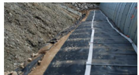
1. Anchor Rods – The arch structure is connected to the GRS soil mass composite with soil anchor rods. The anchor rods ensure the structure maintains shape during backfilling.
