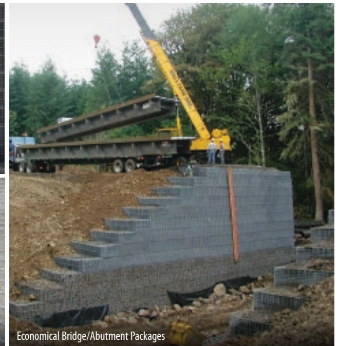
Crusher Wall with natural stone at the face
