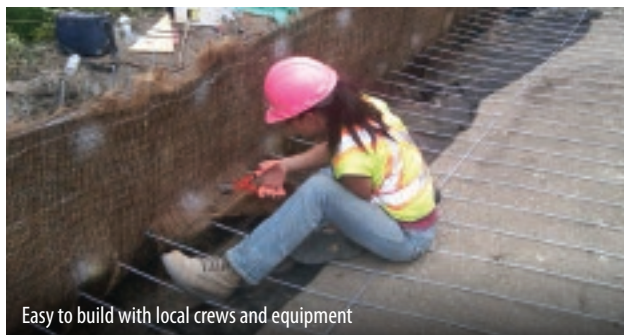
Crusher Wall with geotextile at the face
