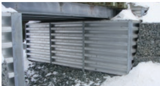
Building Bolt-A-Bin Abutments, Baffin Island, Nunavut
