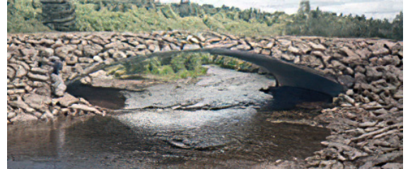
Super•Cor Box Culvert supports forestry road.
