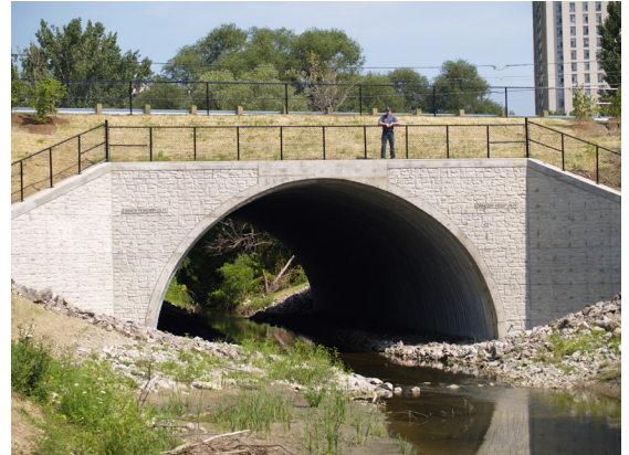
AIL's Super•Cor Arch supports high-traffic Toronto street.
