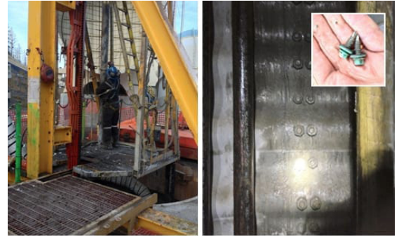
Left: Surface view. Right: Typical circumferential/longitudinal seam; farther up the shaft, self-tapping screws were used (inset).
