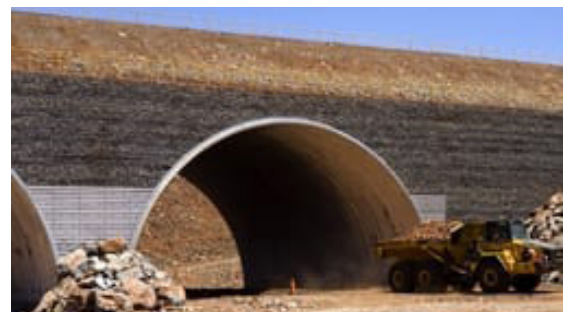
Mining vehicle passes through AIL Super•Cor Arch.
