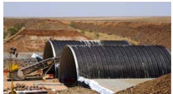
Twin Super•Cor Arches being installed.
