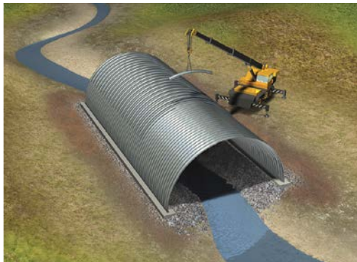
If specified, reinforcement ribs are then added.
