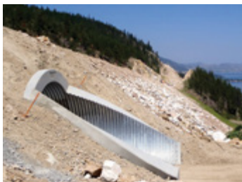
This Bolt-A-Plate® recreational trail and wildlife underpass installed in just eight days. Highway 97, British Columbia.
