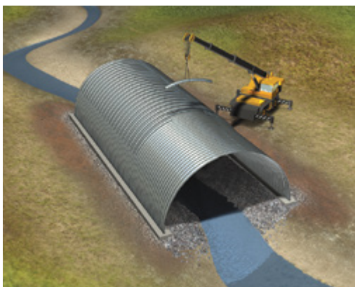
If specified, reinforcement ribs are then added.
