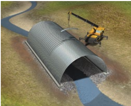
If specified, reinforcement ribs are then added.
