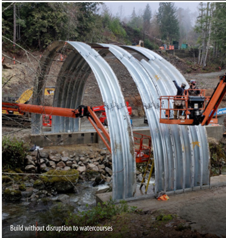
Heavy Haul Road Conveyor Crossing, British Columbia
