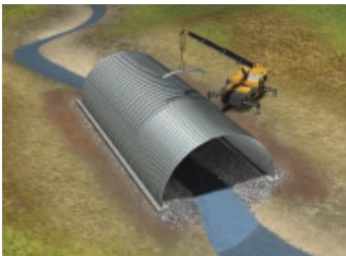
If specified, reinforcement ribs are then added.
