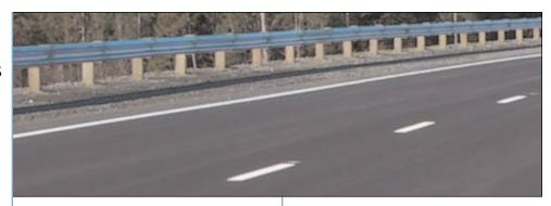
Guiderail is manufactured to the highest specifications (AASHTO M180-18) from 2.67 mm or 3.43 mm steel. All componenets, including nuts and bolts, are hot dip galvanized in a process (CAN/CSA G164M) that provides double the zinc protection of pregalvanized steel. This ensures long service life for all applications.
