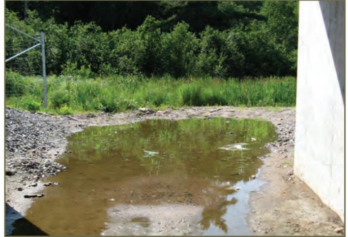
Photo 31. Water accumulation at tunnel entrance. © K. Gunson
