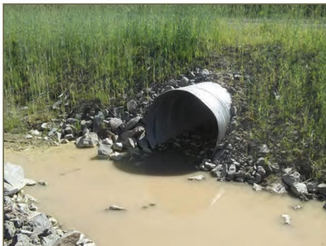
Photo 46. Pooling at culvert entrance that should be avoided at terrestrial wildlife tunnels
