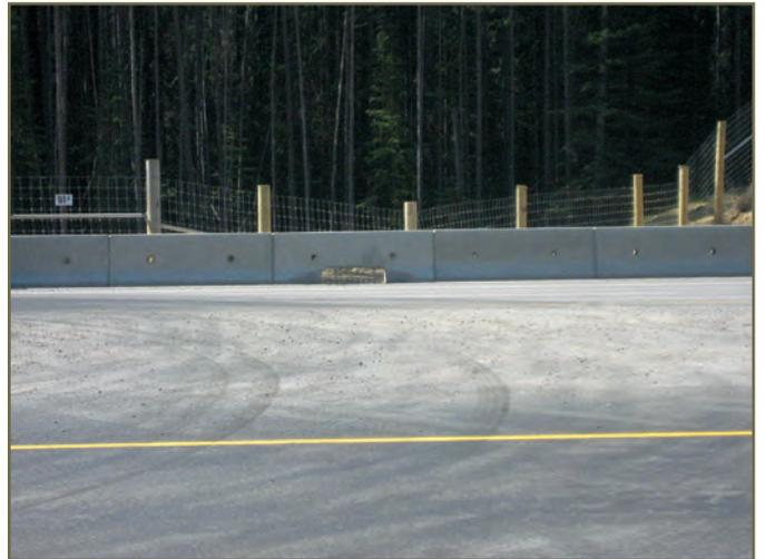
Photo 61. Jersey barrier with gaps at the road surface ©K. Gunson
