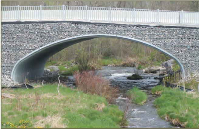
Photo 14. Arched tunnel allowing natural stream crossing. © D. Seburn
