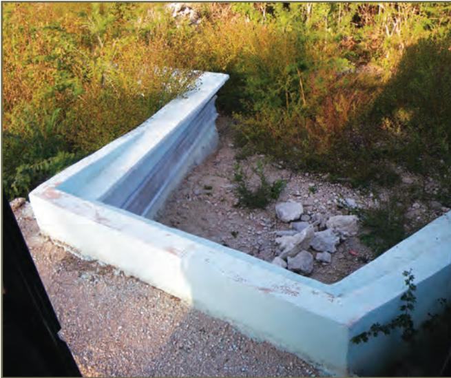
Photo 11. Tunnel with headwalls connected to concrete guide fencing in Cuba.
