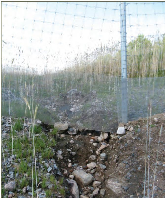
Photo 50. Fence with gap at bottom due to erosion from water draining under fence © K. Gunson
