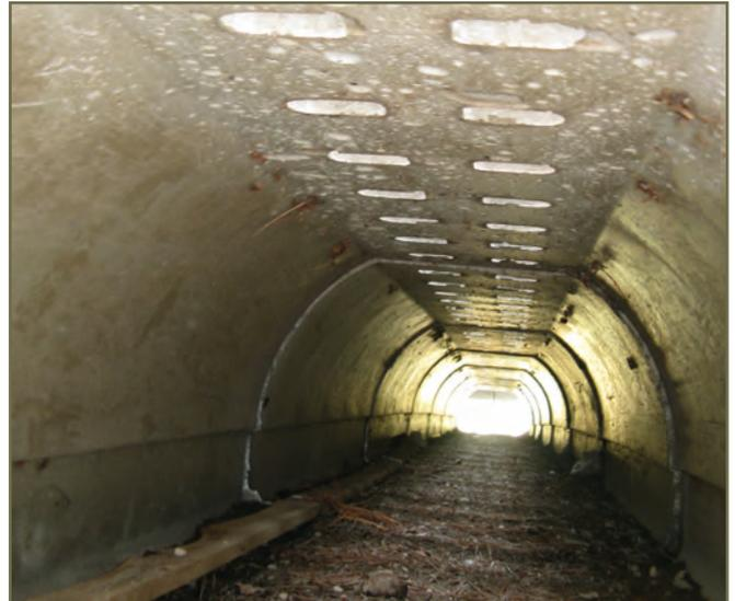
Photo 8. ACO open-top tunnel allowing light into tunnel. © Kari Gunson
