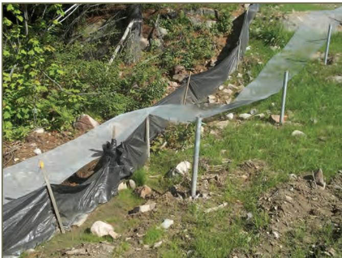
Photo 63. Temporary fencing installed prior to installation of more permanent fencing along highway 69, note permanent fencing completed in Photo 48. © W. Kowbasniuk
