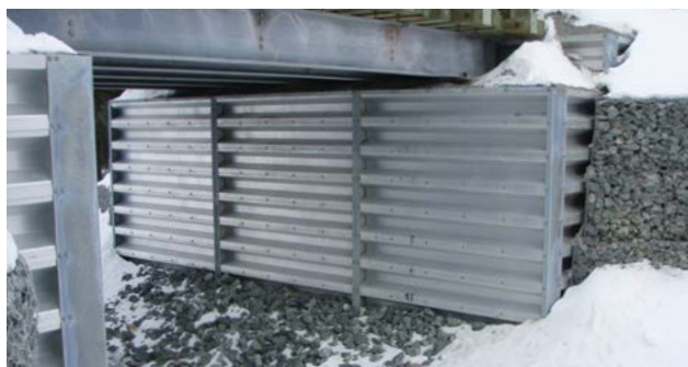
Building Bolt-A-Bin Abutments, Baffin Island, Nunavut
