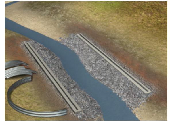
The first arch segment is completely assembled on the ground.
