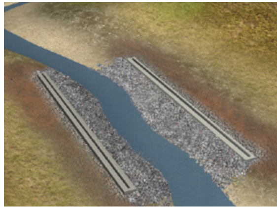
Precast or cast-in-place concrete footings are set over the prepared site.
