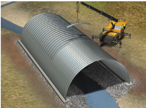
If specified, reinforcement ribs are then added.
