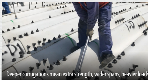
Completing first ring in Ultra-Cor® plate assembly.
