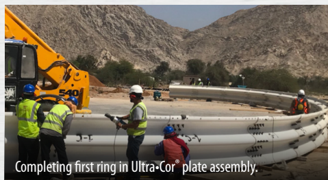
Lifting of first Ultra-Cor® ring assembly.
