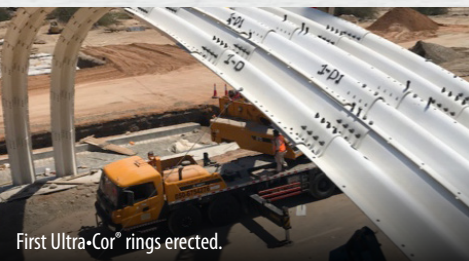
Beginning of Ultra-Cor® plate assembly.
