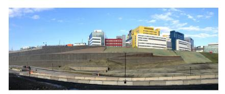
Our six-wall project featured 3 m x 1.5 m precast panels in eight different horizontal pattern configurations. The larger size panels required extra care in shipping and handling. A specialized, antigraffiti coating was applied by others after installation.
