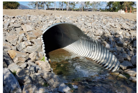
Popular Pipe Arch shape is wider at the bottom
