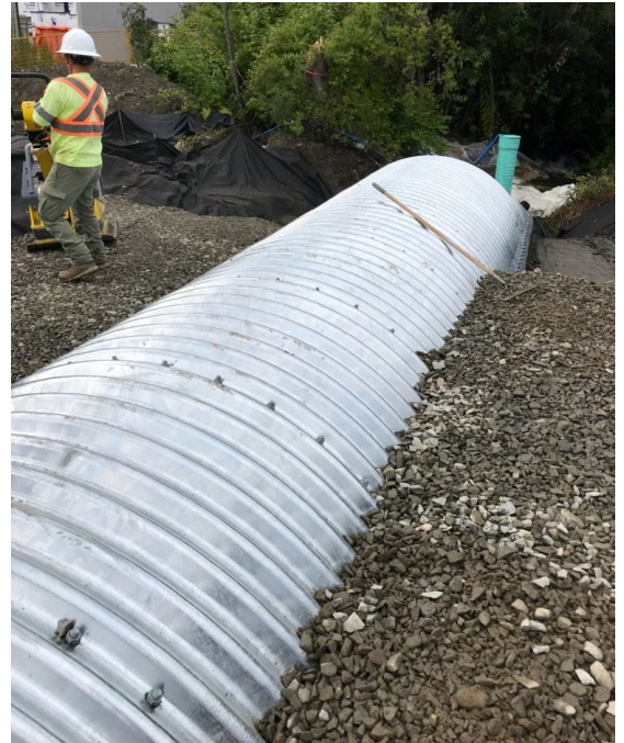
Backfilling of first half of two-stage installation
