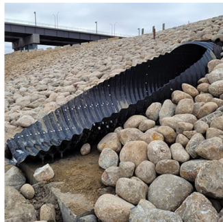
Left: Before photo of the installation site. Right: New culvert installed in stabilized embankment.
