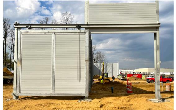
The noise barrier wall needed to navigate around some underground utilities and included two large sliding gates that were each 16' tall x 15' wide.
