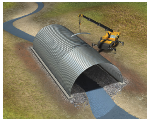
If specified, reinforcement ribs are then added.
