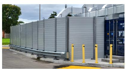
The noise barrier wall was flange-mounted to the curved concrete pad and also supported a curved quardrail.
