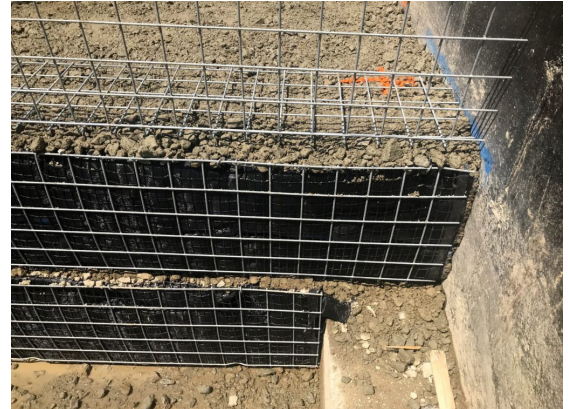
First two lifts of temporary wire wall
