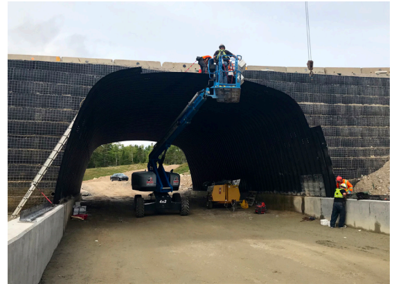
Temporary wire wall on median side of phase one
