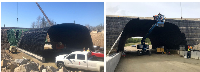
Phase one plate assembly nearing completion (l) and beginning of phase two assembly (r)
