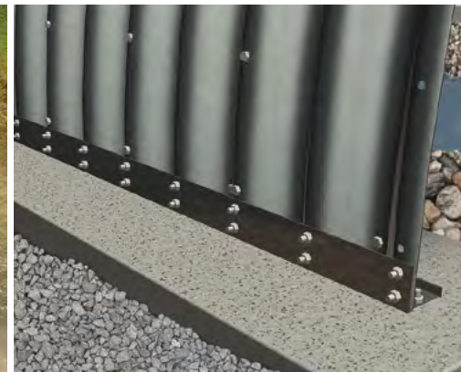
The segments bolt into base channels, integrated into the concrete.
