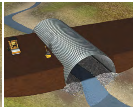
Layers of engineered backfill are added in sequential lifts.
