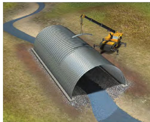
If specified, reinforcement ribs are then added.
