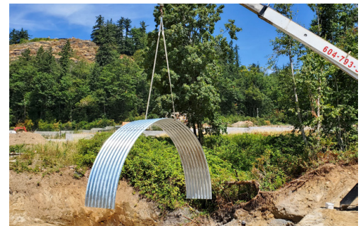
First section being placed for Bolt-A-Plate culvert
