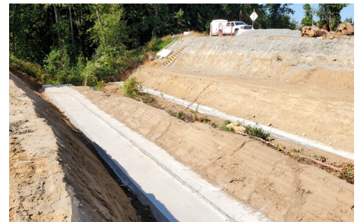
Prepared foundation footings for Bolt-A-Plate culvert
