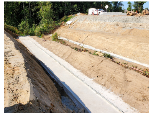
Prepared foundation footings for Bolt-A-Plate culvert
