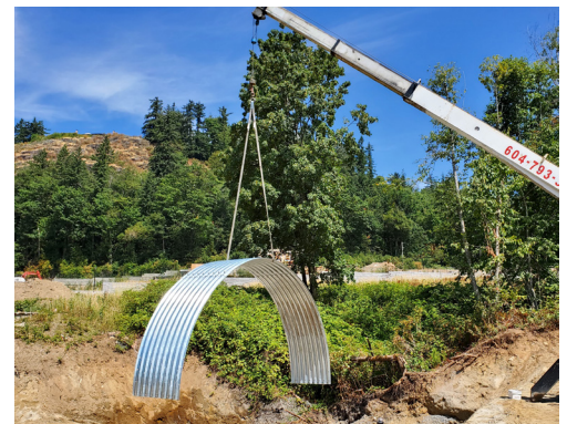
First section being placed for Bolt-A-Plate culvert
