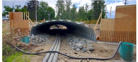
Climate change washout resilience: wider span, scour protection and concrete headwalls
