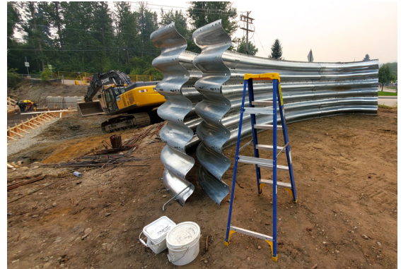
Box culvert sections pre-assembled on-site
