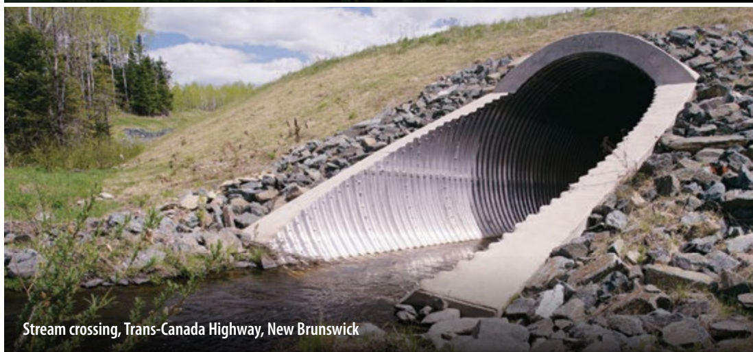
Stream crossing, Town of Plympton-Wyoming, Ontario
