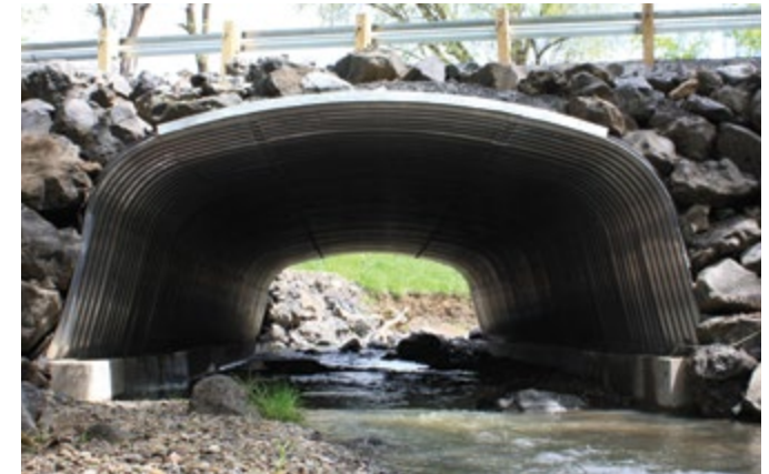
Stream crossing, Town of Plympton-Wyoming, Ontario
