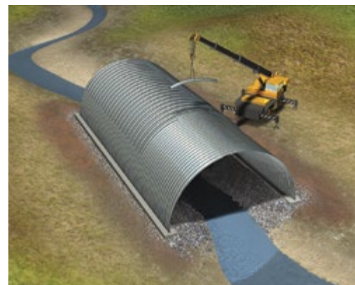
If specified, reinforcement ribs are then added.
