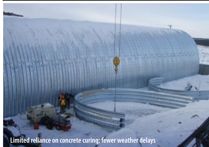
Heavy Haul Road Crossing, White Horse Creek, Northern Alberta
