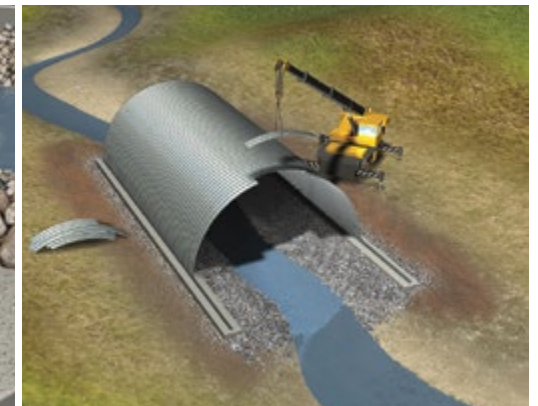
Plates then attach individually to make up other arch segments.
